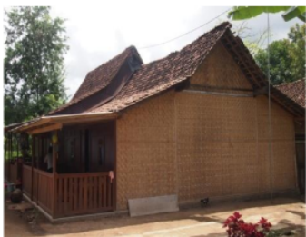
Figure 1 The Using House in Kemiren Village with Bamboo Plaster
