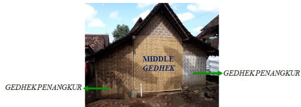
Figure 4. Using's House Walls
