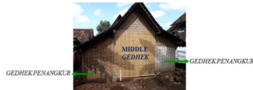
Figure 4. Using's House Walls
