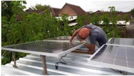
Gambar 2. Instalasi Panel Surya Gazebo 1
