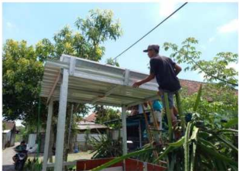
Gambar 3. Instalasi Panel Surya Gazebo 2
